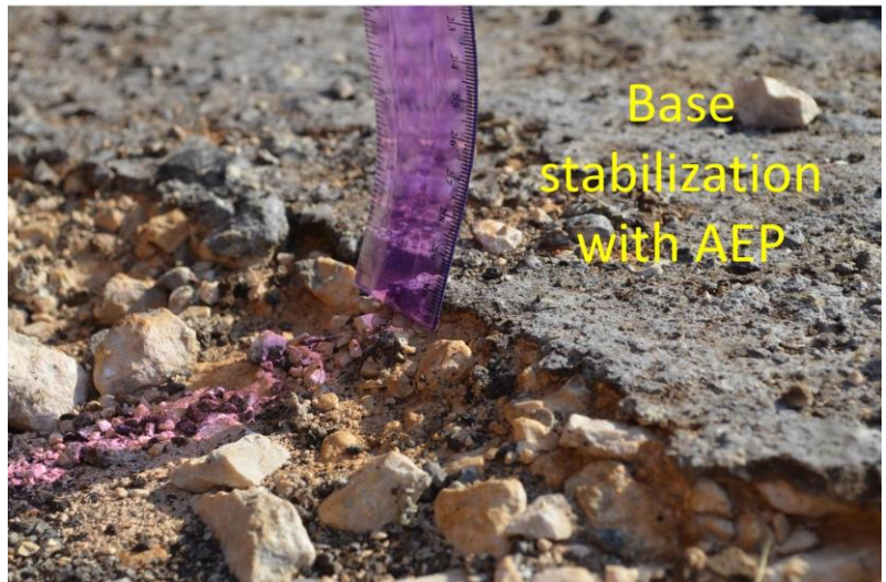
AEP Prime coat in Florence, Texas: Less than 1 inch penetration
