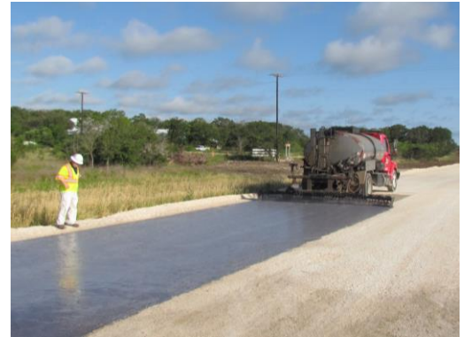
Terra Prime TM application in Florence, Texas
