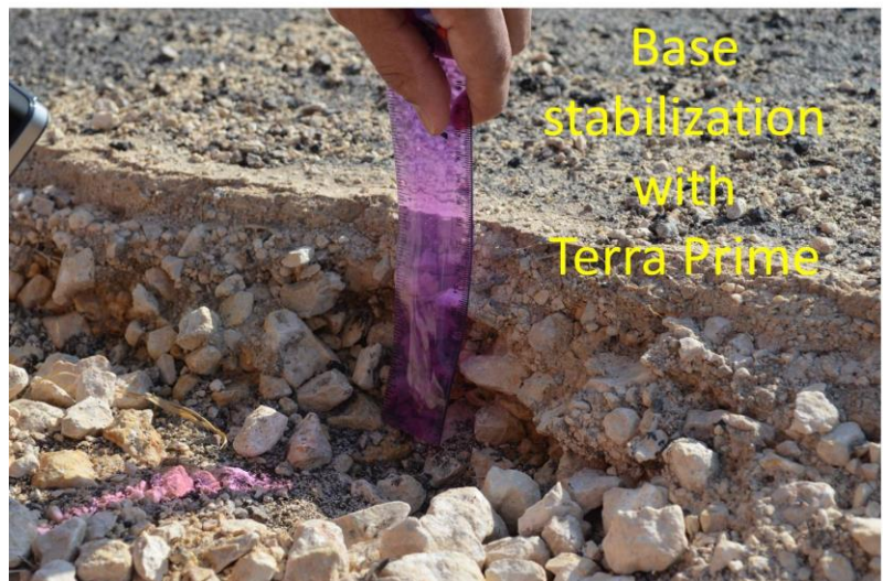
Terra Prime™ in Florence, Texas – More than 4 inches penetration
